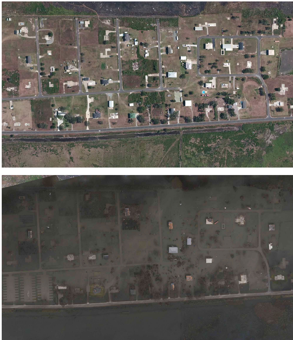
Figure 12. Near Cameron, Louisiana before (top) and after (bottom) Hurricane Laura. Images courtesy of NOAA National Ocean Service.
