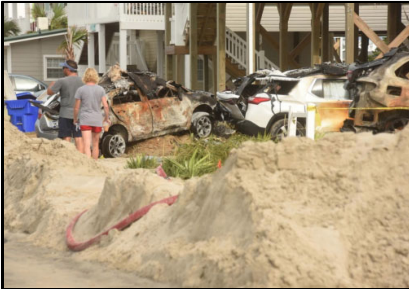
Figure 14. Storm surge damage in Brunswick County, NC. Photo credit Town of Southport.
