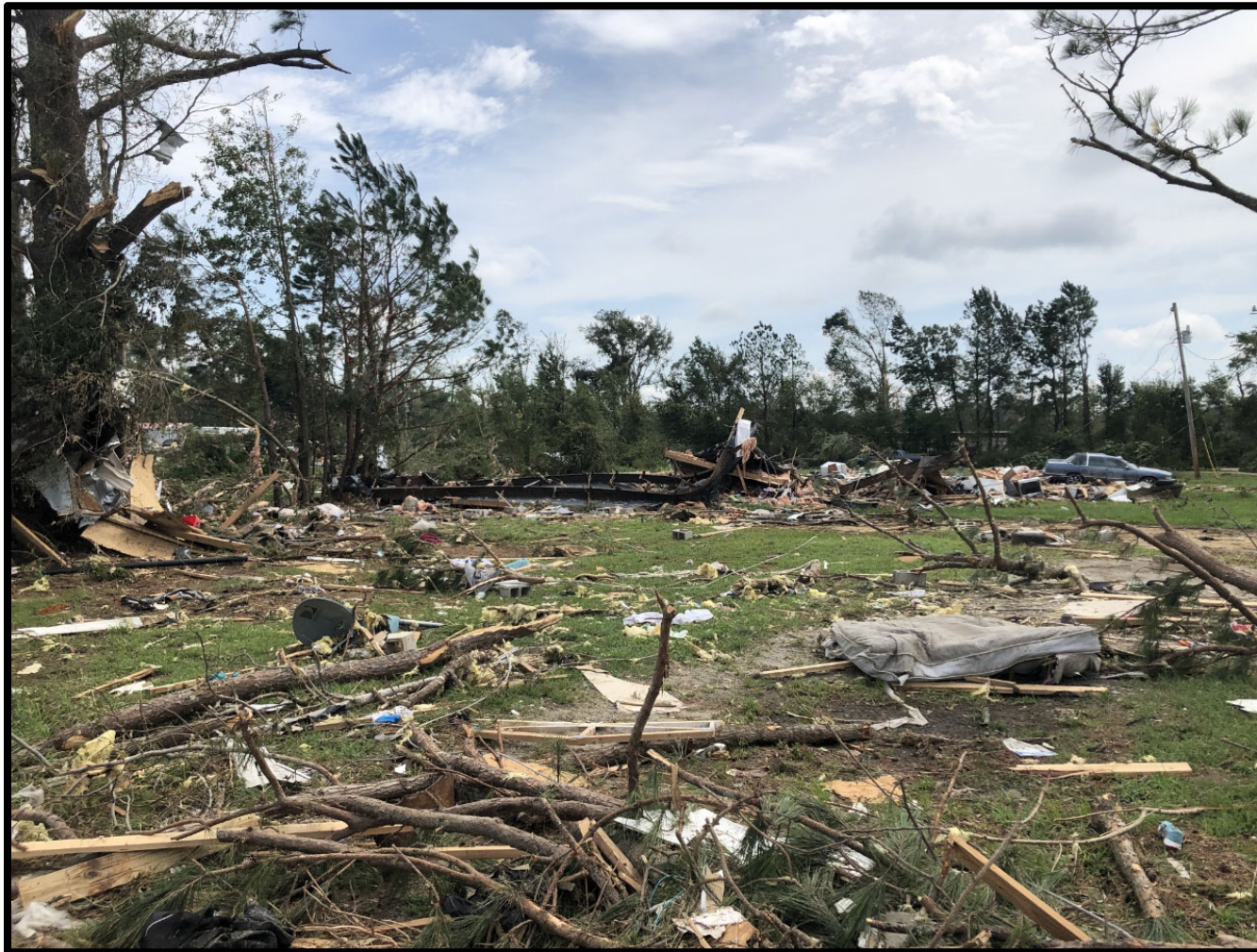
Figure 13. Tornado damage in Bertie County, NC. Photo credit NWS WFO Wakefield, VA.
