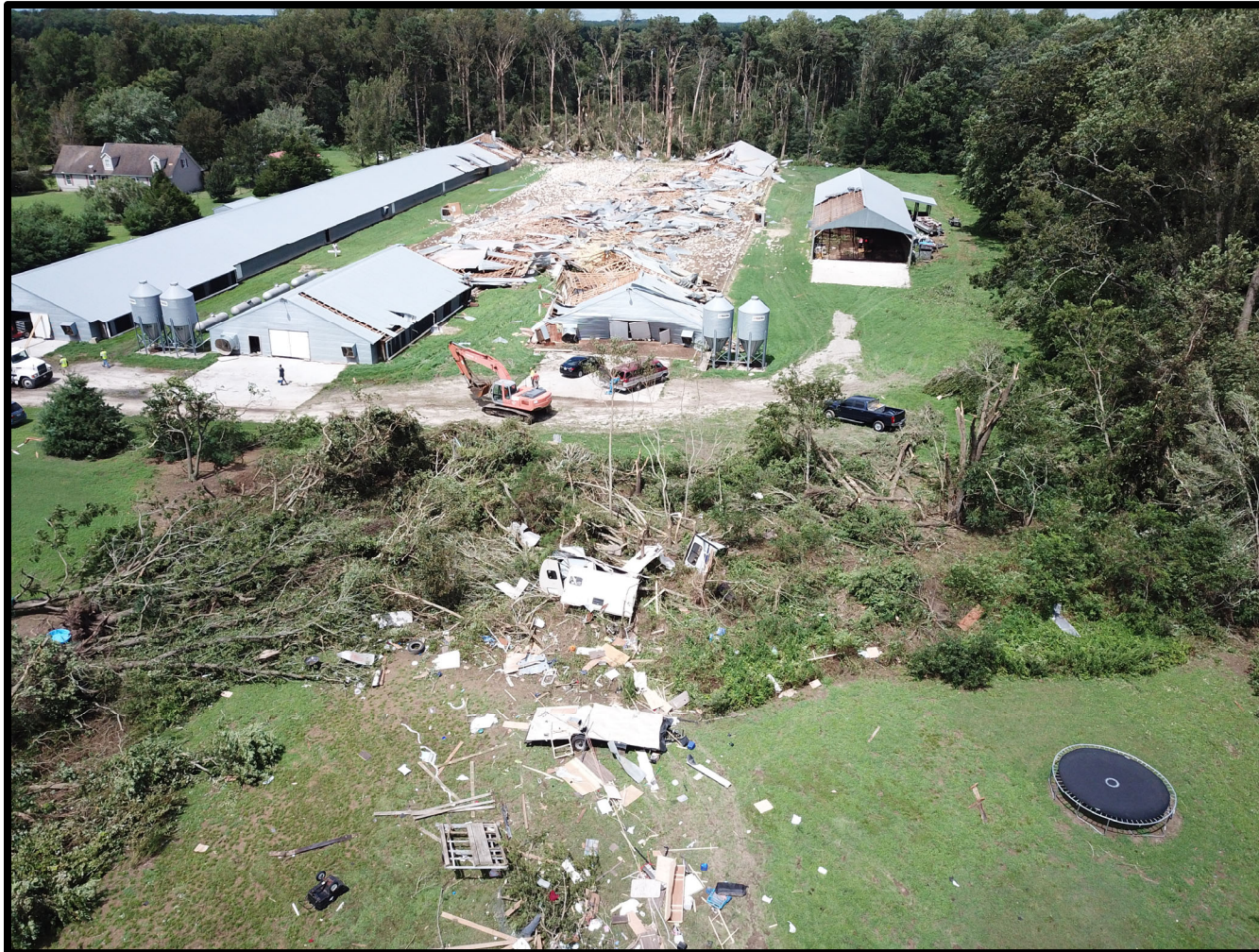
Figure 17. Tornado damage in Stockton, MD. Photo credit NWS WFO Wakefield, VA.
