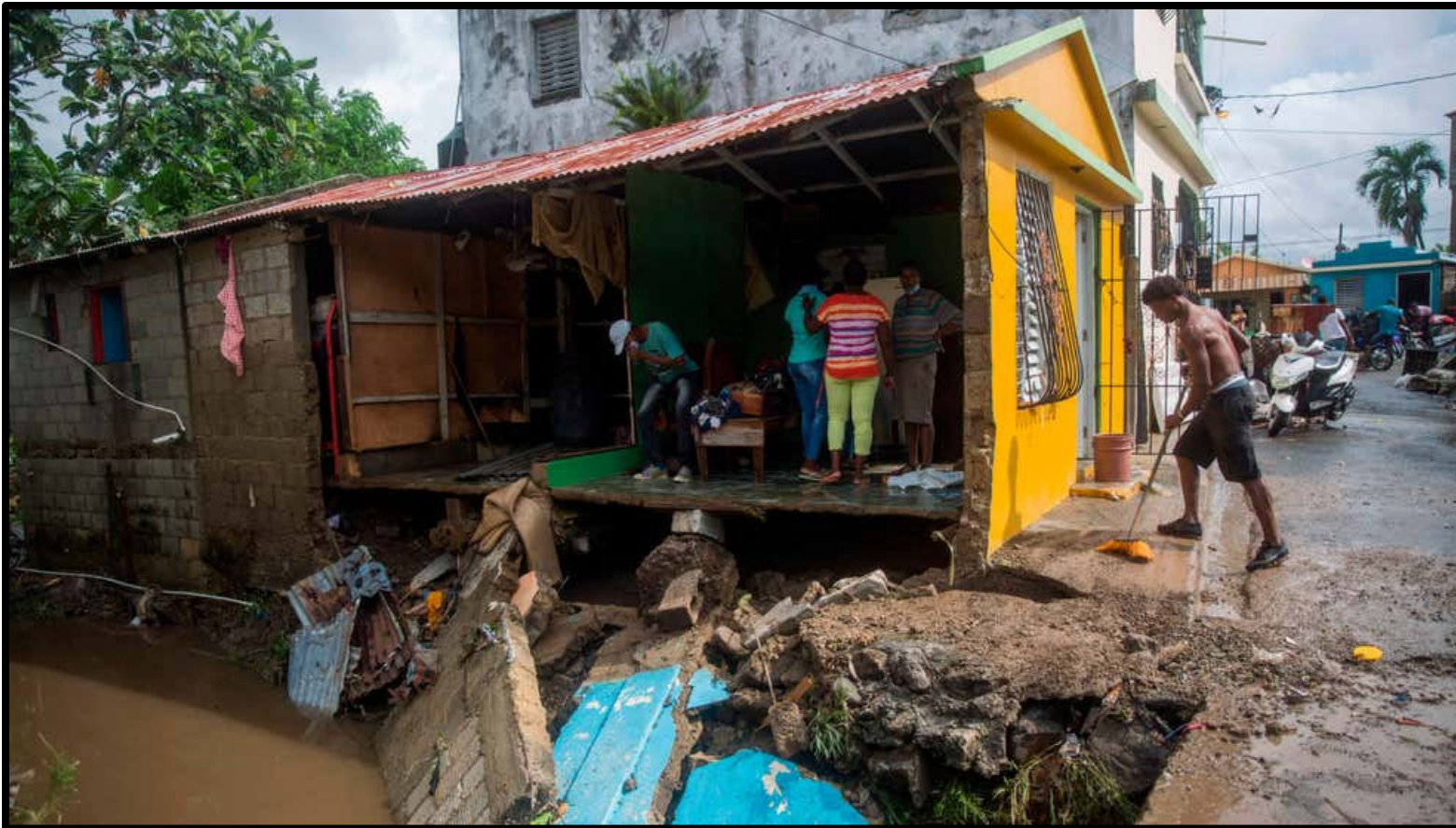
Figure 7. Isaias' flash flooding damage in the Dominican Republic. Photo credit Getty Images.
