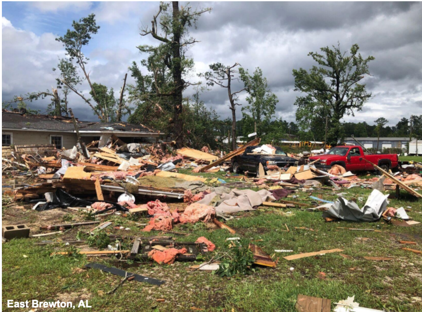
Figure 7. Damage associated with an EF-2 Tornado in East Brewton, AL. Image via Fox10 News ( https://www.fox10tv.com/news/alabama/ts-claudette-brings-tornado-damage-to-southern-alabama/article_b974600c-d16a-11eb-8446-674d90b6b3dd.html ).
