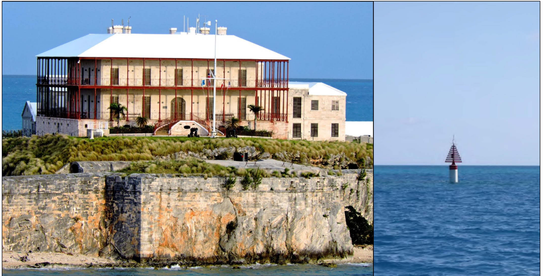
Figure 12. Commissioner's Point, Bermuda, observation location viewing west (left panel). Anemometer equipment located on the top of the roof could have produced accelerated and unrepresentative wind speeds due to the Bernoulli Effect created by air flowing over the hipped-roof on the Commissioner's House structure. Crescent Beacon NAVAID (right panel) located approximately 8 n mi northwest of Bermuda.
