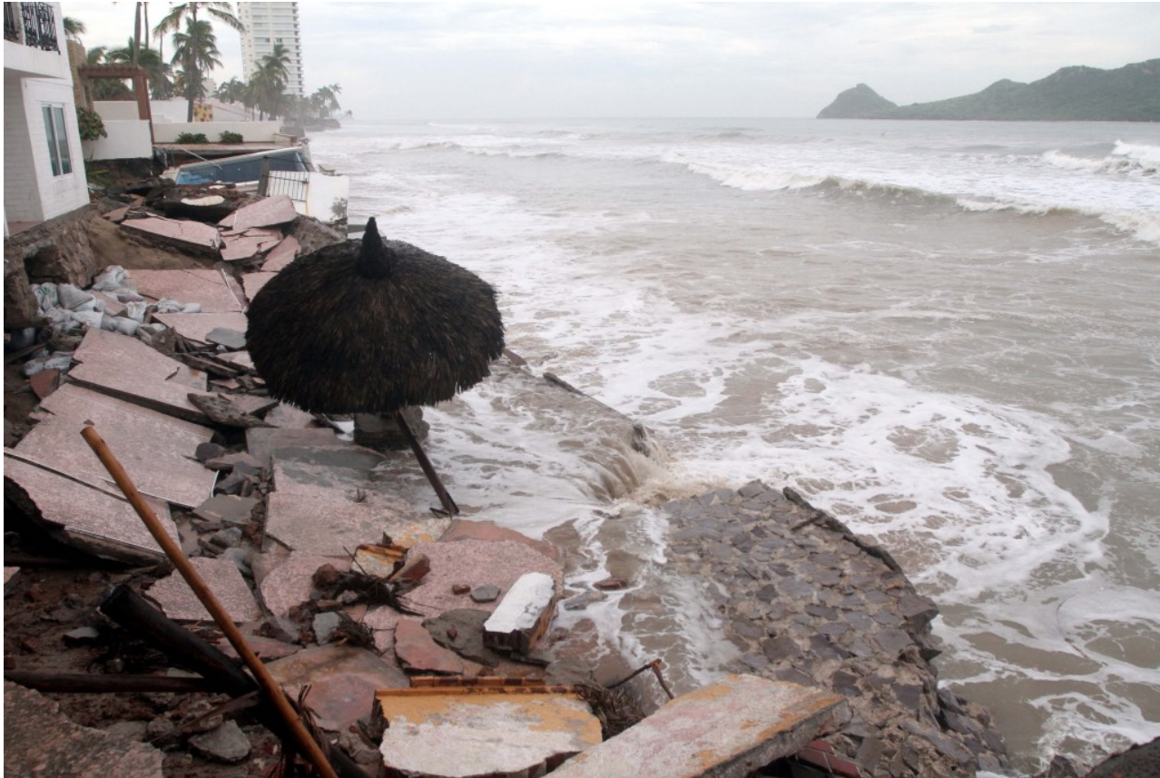
Figure. 5 Impact of high waves associated with Hurricane Norbert in the port of Mazatlan, Mexico. Photo provided by the University of Guadalajara, Mexico.
